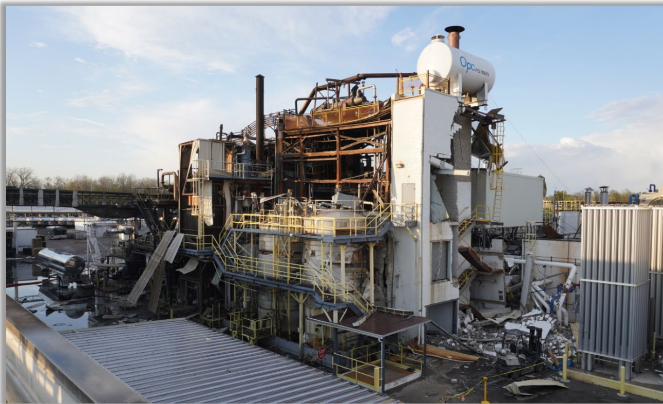
Figure 1. Resin plant the day after the incident. (Credit: CSB)
