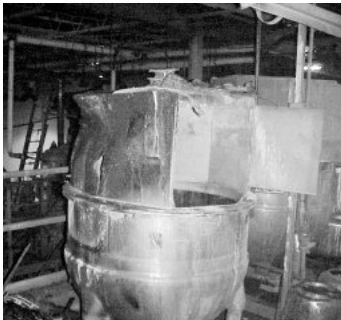
Figure A-2. Silver nitrate reactor on mezzanine 1 with open tank door (following explosion and fire).
