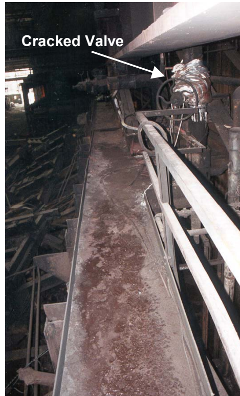
Figure 9. Elevated walkway looking south (note absence of handrail on left side).
