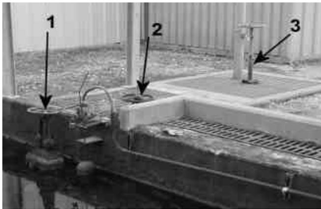
*Figure 5. Oil pit control valves.*
