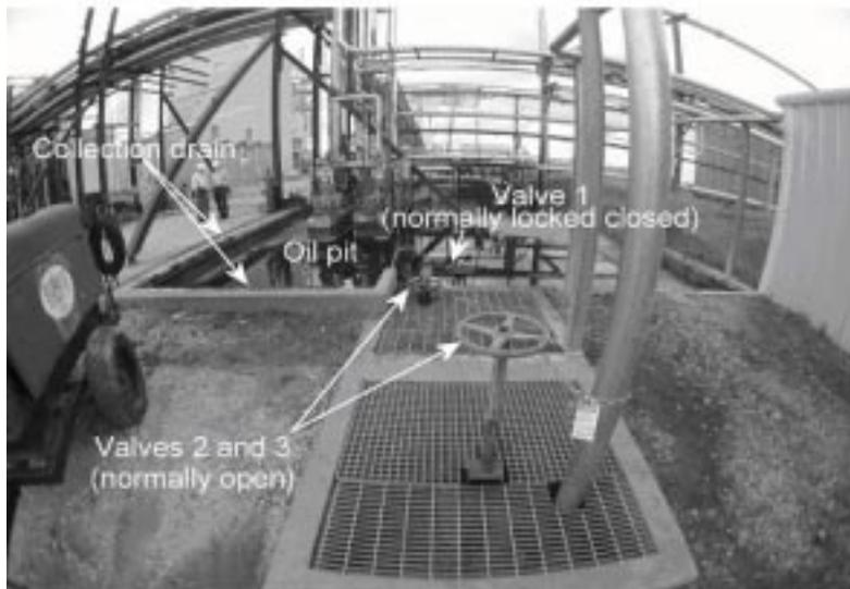
Figure 4. Oil pit and adjacent tank truck unloading station.
