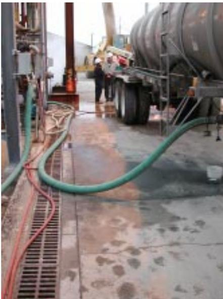
Figure 3. Collection drain next to tank truck unloading station.
