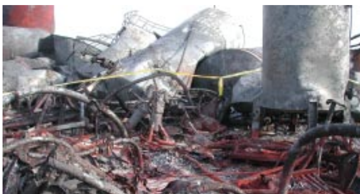
Figure 7. Collapsed blend tanks located near warehouse 1.
