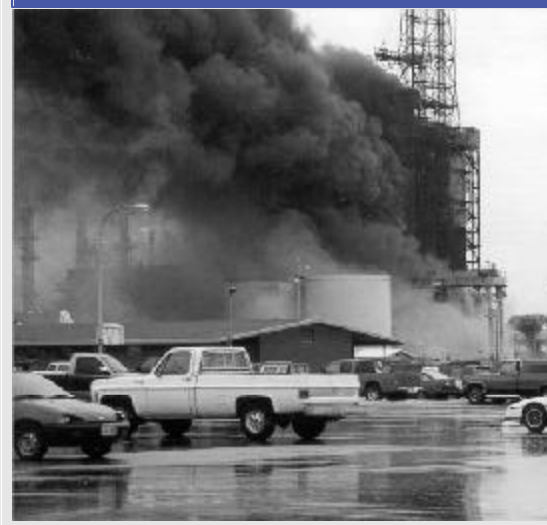
● Figure 1. Equilon Enterprises oil refinery fire.
