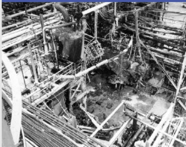
● Figure 3. Site of ruptured reactor, CONDEA Vista Company detergent alkylate plant.
