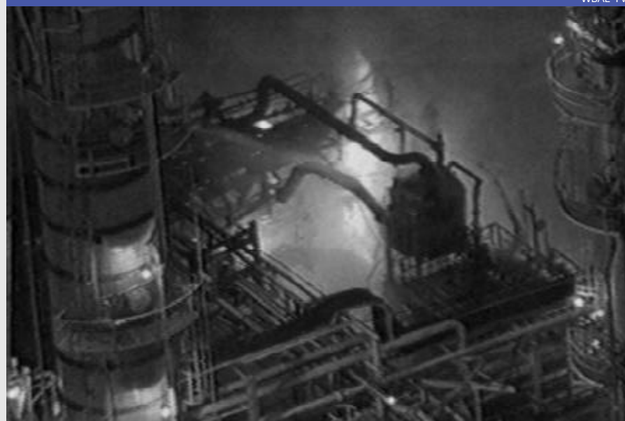
● Figure 4. CONDEA Vista plant fire.
