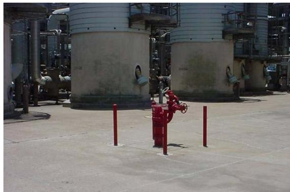
**Figure 9. Protection of fire fighting equipment.**
