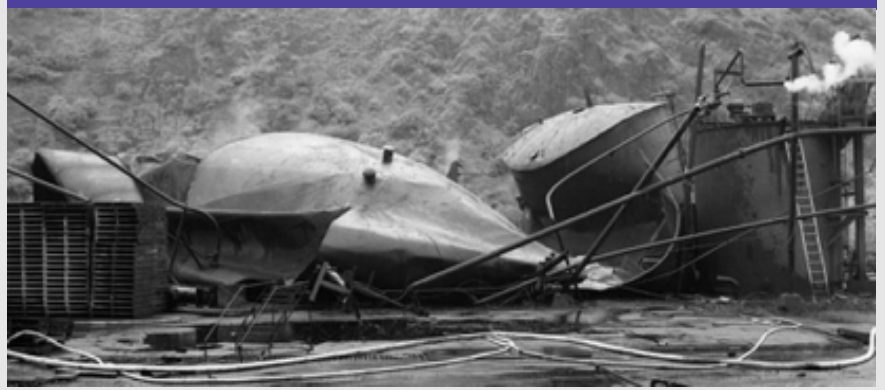
● Figure 8. WESTVACO paper mill tank failure.
