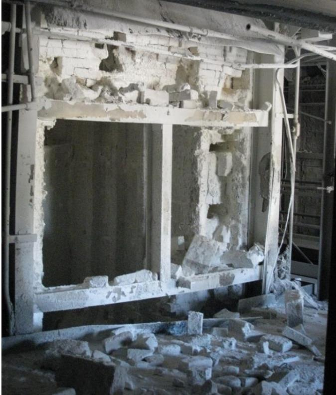
This photograph shows the combustion chamber wall of column B, and the site of the explosion, the pressure relief panels being blown out into the workplace.
