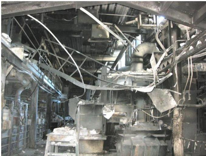
This photograph shows a typical scene within the plant after the explosion and fire. It is a general view showing damaged plant and equipment, all covered with a zinc oxide ash.
