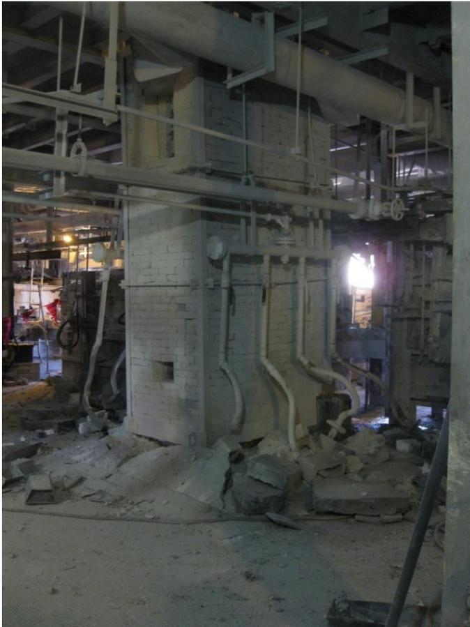
This photograph shows the reflux tower after the explosion. The trays in the combustion chamber have collapsed but the reflux tower is largely undamaged, having dropped a few feet such that the framework for the reflux section insulation was sitting on the combustion chamber roof.
