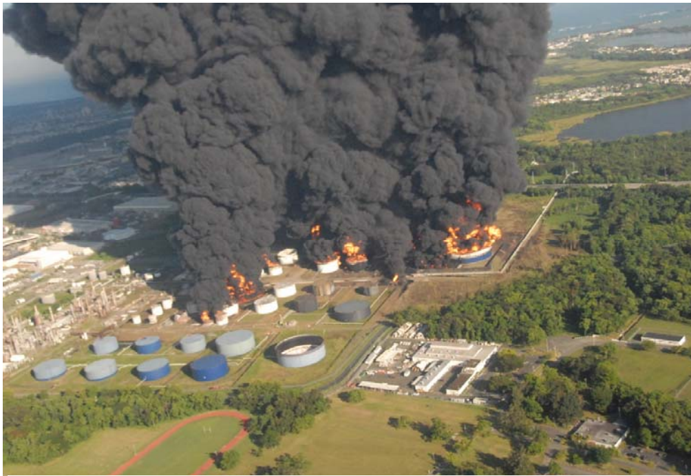
Figure 5: CAPECO multiple tank farm fire, October 23, 2009.
