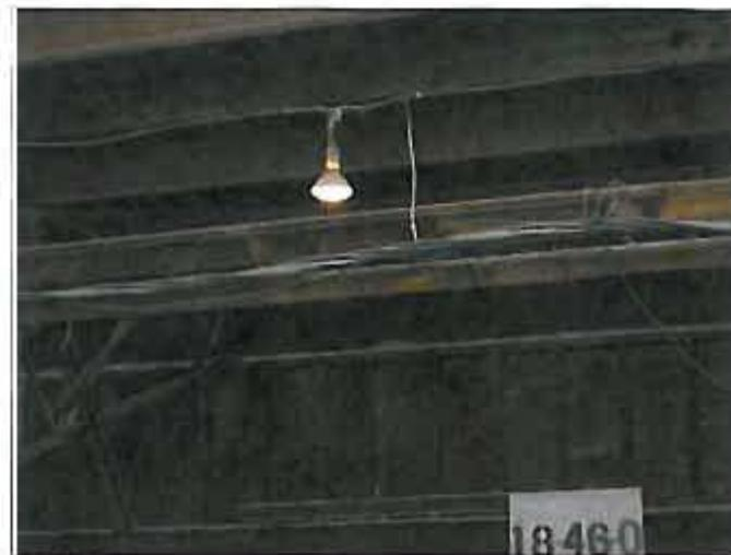
Figure 53. Exposed 440-Volt Electrical Wiring Identified in 2007 Survey
