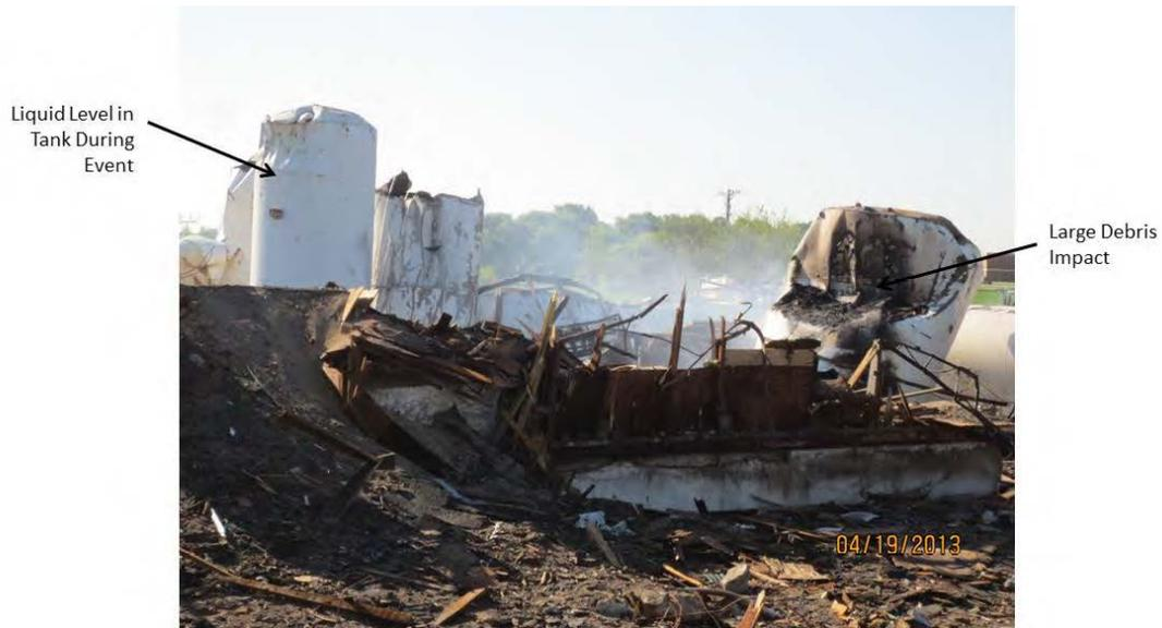
Figure 16. Liquid Fertilizer Tank Damage (Source: CSB)
