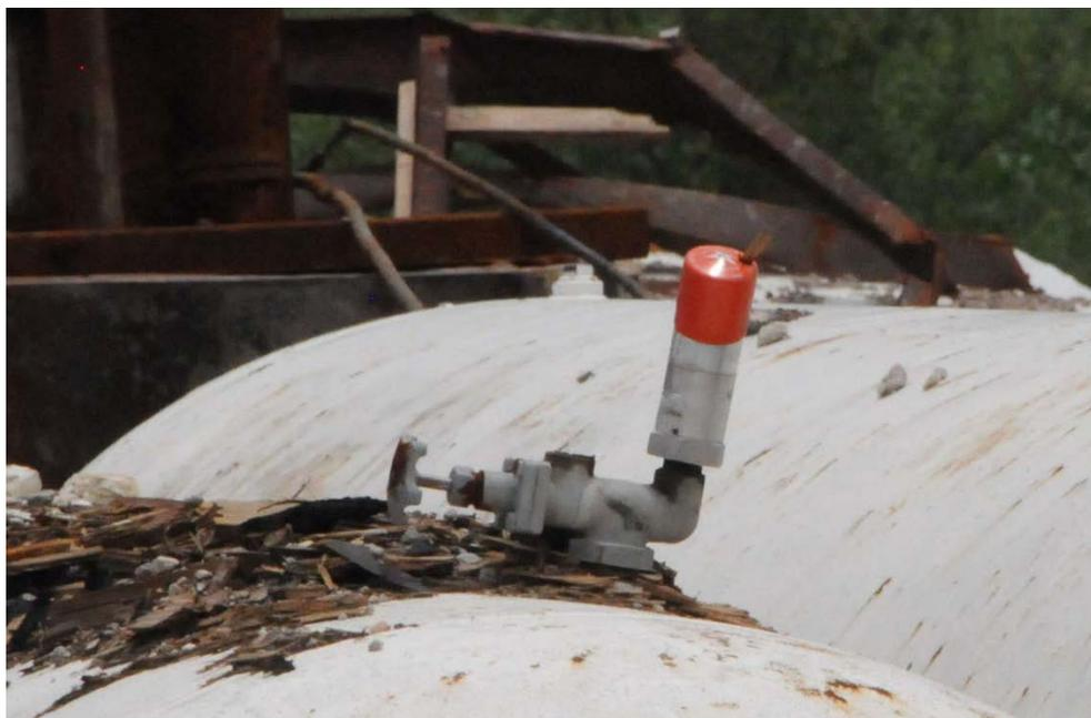
Figure 21. Anhydrous Ammonia Tank PRV, Post-Incident (Source: CSB)
