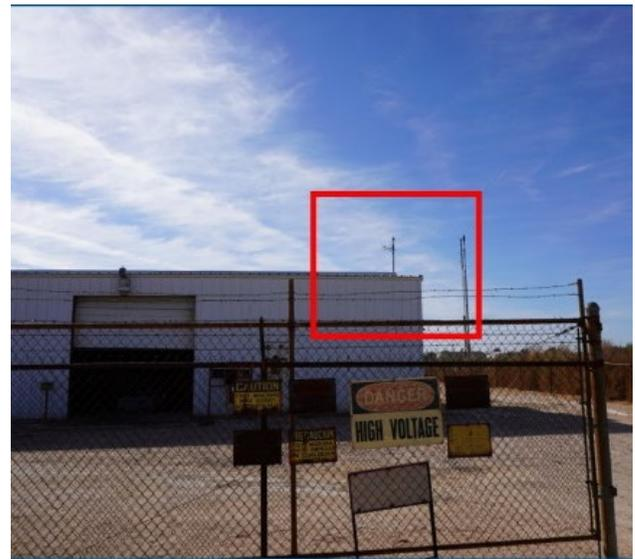
**Figure 16.** Light designed to illuminate when a dangerous concentration of H<sub>2</sub>S is detected. (Credit: CSB)
