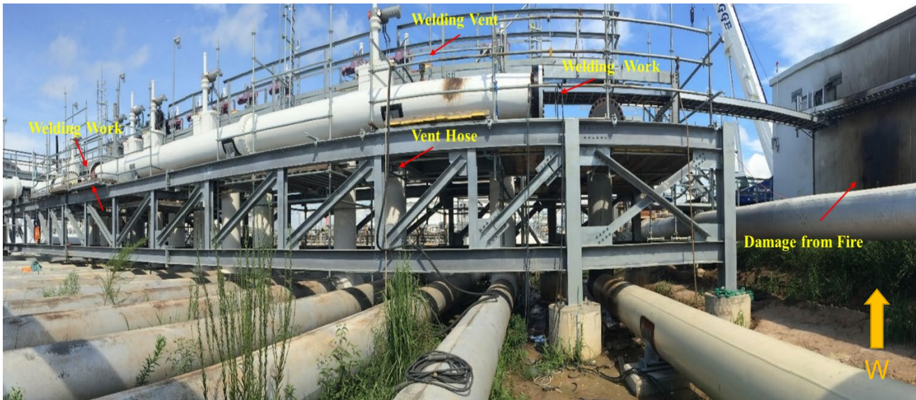
Figure 17. West-facing view of the section of piping where welding work was ongoing (on the north end) at the time of the incident. (Credit: CSB)
