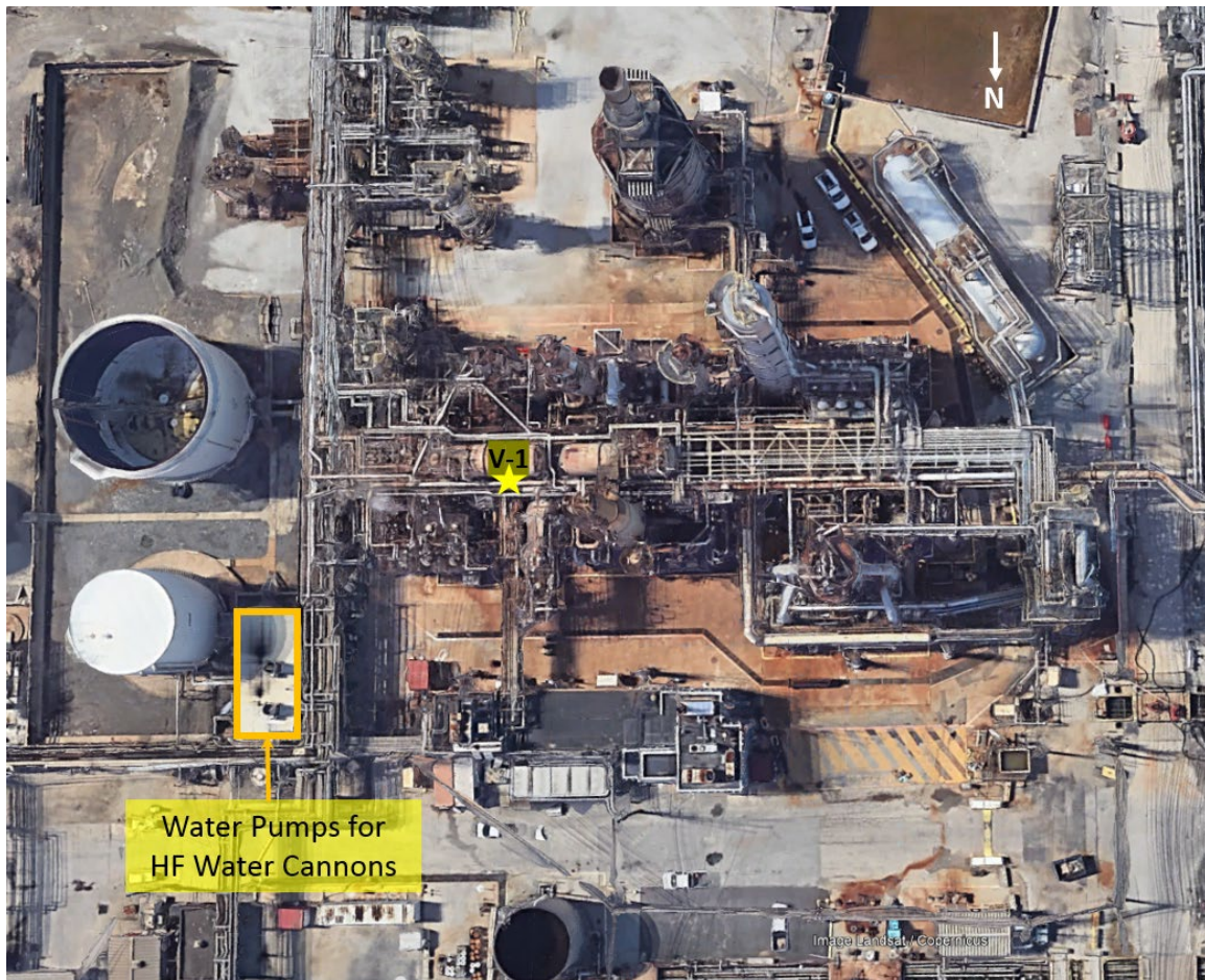
Figure 10. Location of (1) the water pumps that fed the hydrofluoric acid mitigation water cannons (yellow rectangle), and (2) the location of the ruptured elbow from which the process release originated (yellow star). (Credit: Google Earth with annotations by CSB)
