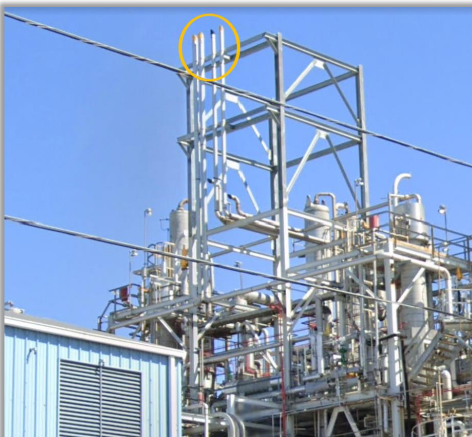
Figure 25. Post-incident Emergency Pressure-Relief System Modifications. (Credit: Google Maps annotated by CSB)
