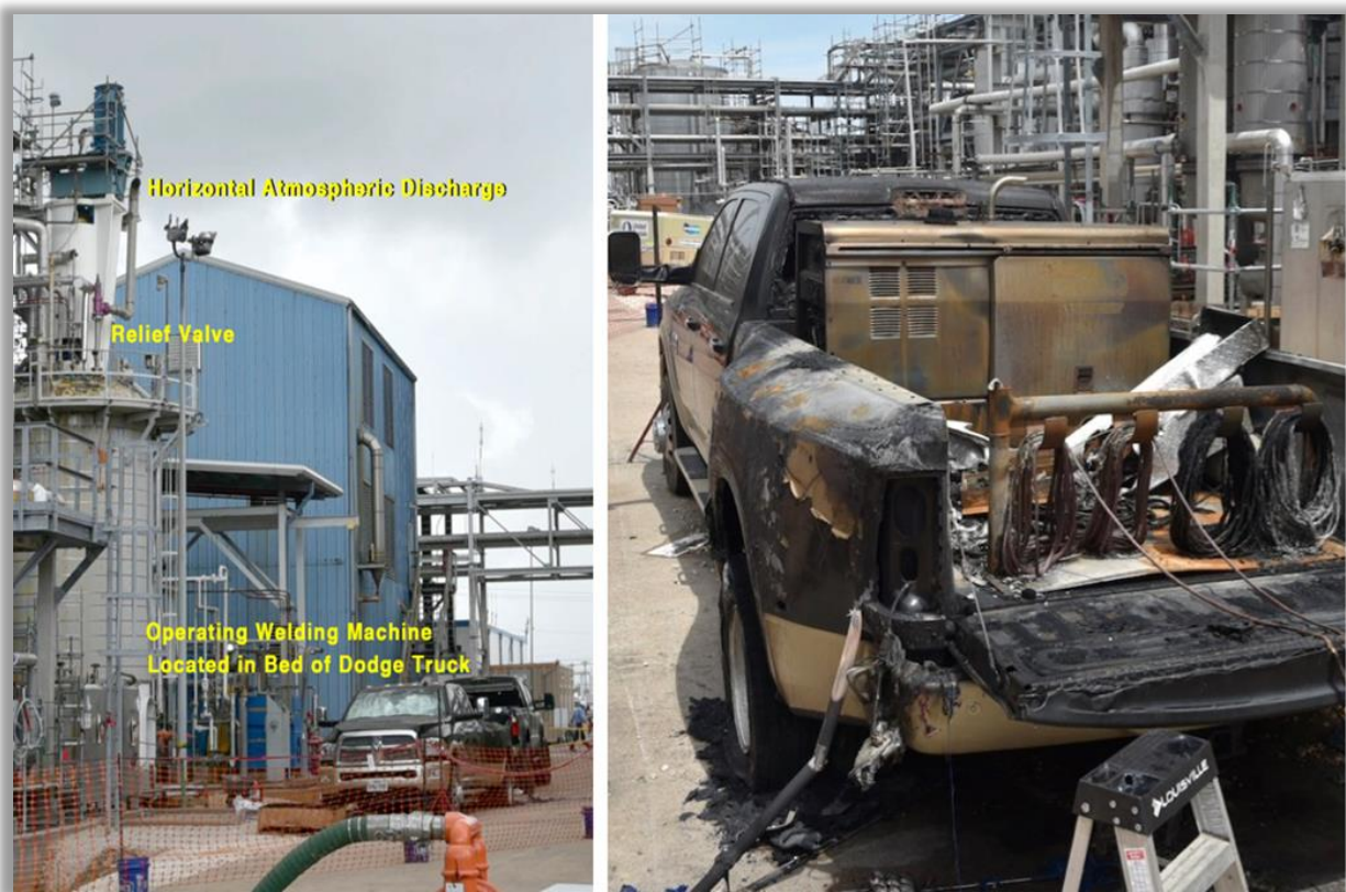
Figure 16. Likely Ignition Source. (Credit: CSB [23])
