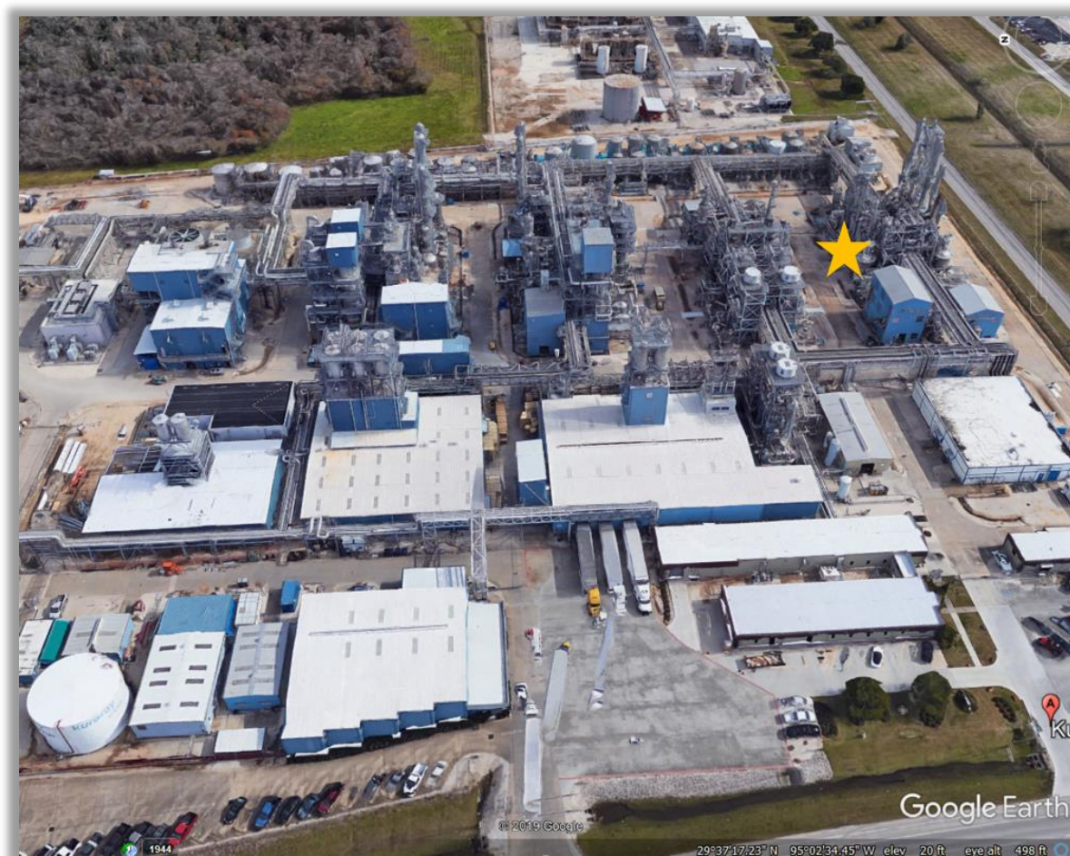
Figure 2. Kuraray EVAL Plant. (Credit: Google Earth)
