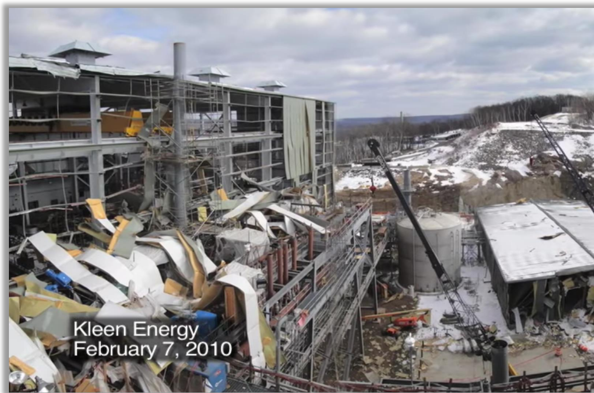
Figure 29. Explosion Damage at Kleen Energy. (Credit: CSB [84])
