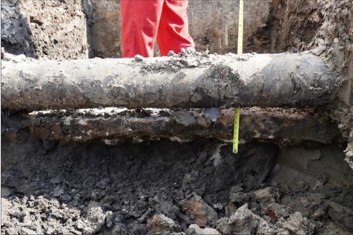
Photo 23: Containment wall footing and underside of footing
