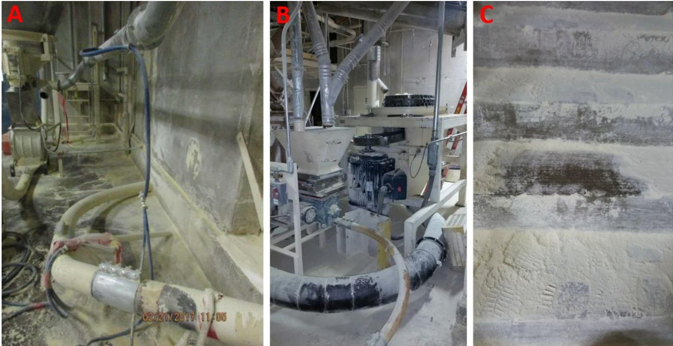
**Figure 58:** Examples of fugitive dust accumulations, (A) approximately three months before the incident, (B) approximately two weeks before the incident, and (C) less than 24 hours before the incident. (Credit: Didion)
