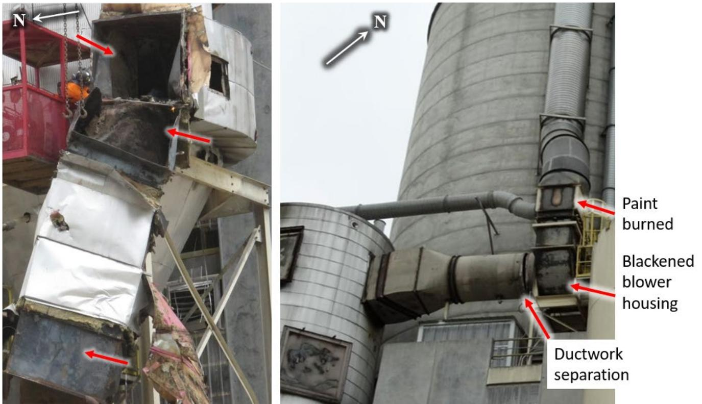
**Figure 32:** Examples of Dry Grit Filter ductwork and blower damage (red arrows). Inlet duct blackened (shown during demolition, left) and exhaust to atmosphere, including blower (right). (Credit: left, Didion with annotations by CSB; right, CSB)
