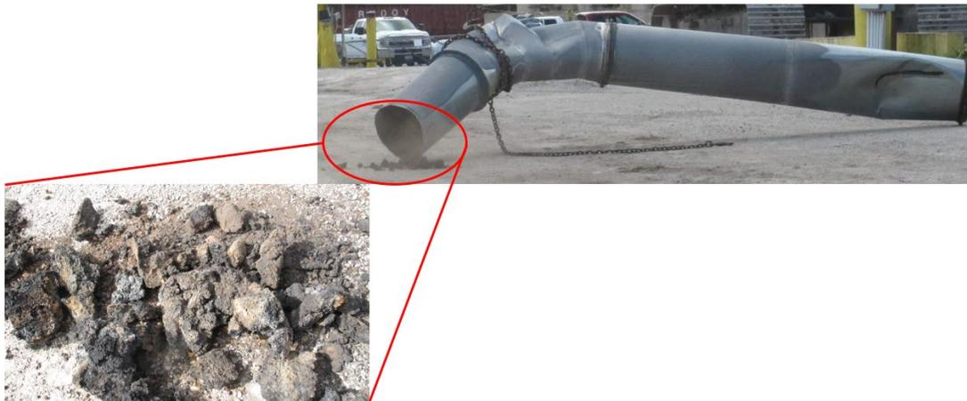
**Figure 48:** Dry Grit Filter supply ducting post-incident (right) with corn product accumulation (inset). Material fell out of ductwork during demolition. (Credit: CSB, adapted from EFI)
