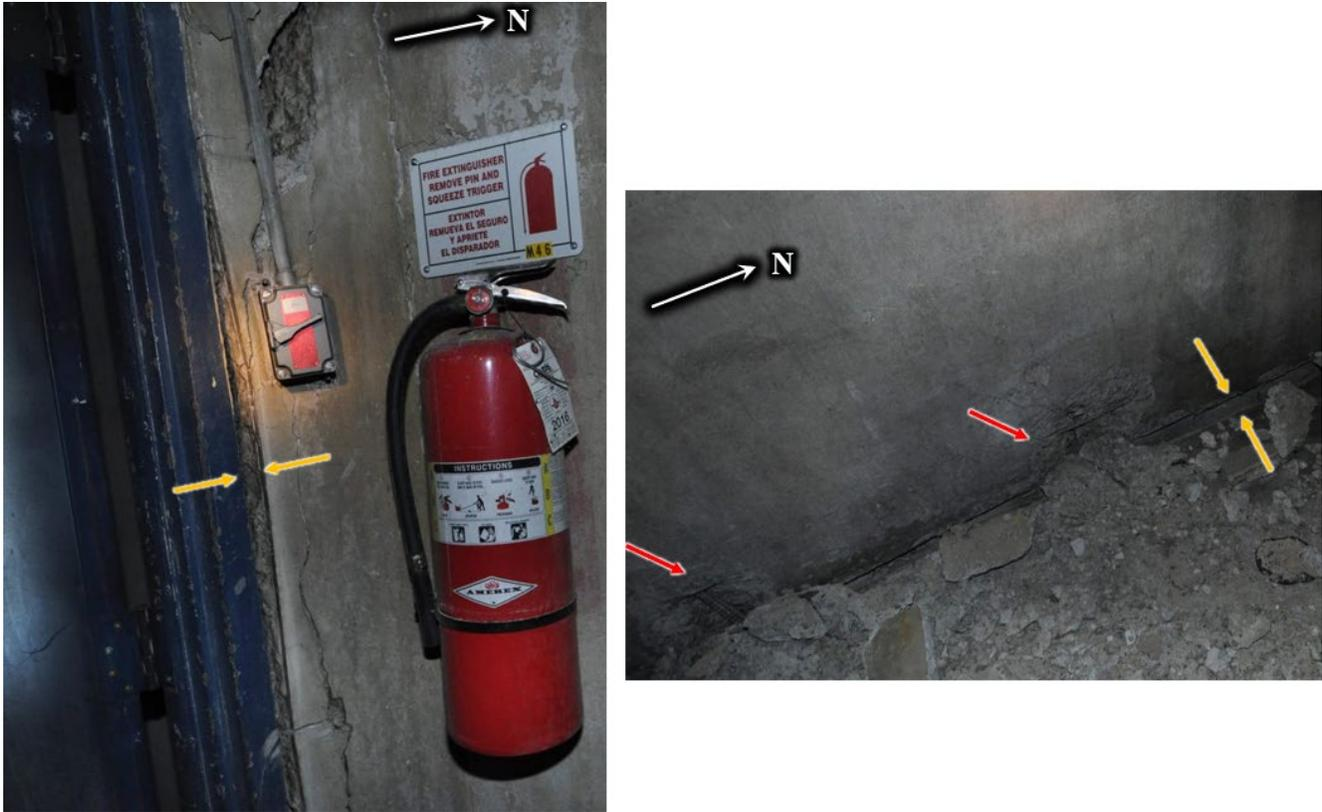
**Figure 41:** 4A structural damage. Wall bowed and separated from door frame (left, at arrows) and wall separated from floor (right, at orange arrows). Note that wall displacement caused concrete damage, exposing rebar (red arrows). (Credit: CSB)
