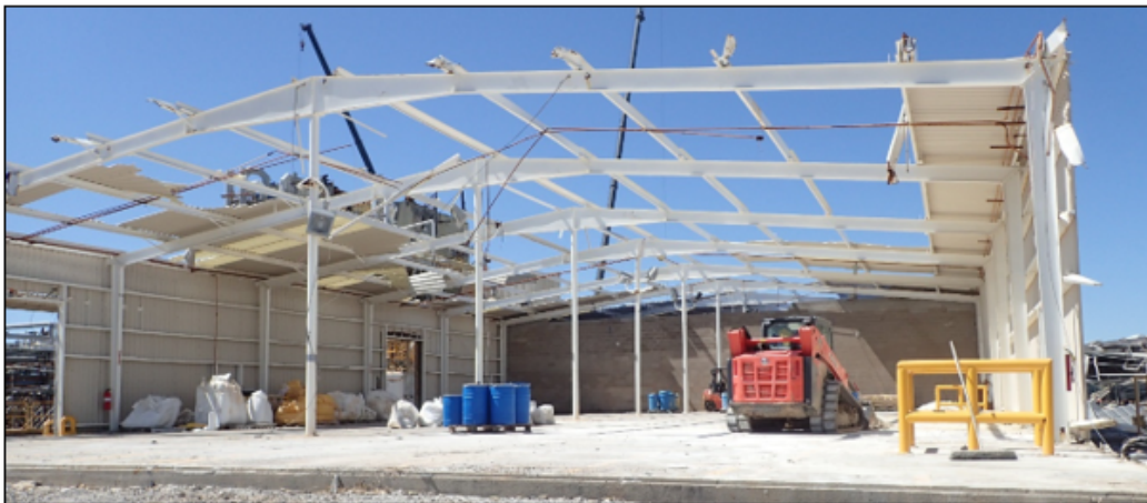
Eastern bay of south FGW, looking SW. Wrecked framing has been removed (Atlas, 9/29/2020)
