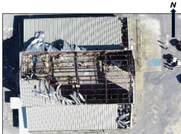
A-Z Building (Atlas UAV, 9/30/2020)
