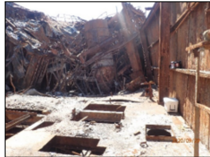
4 th floor level, from north stair (Atlas 9/29/2020)
