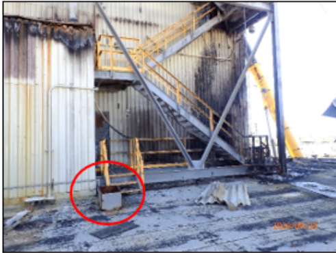
Roof opening at broken duct, Low Bay roof north of High Bay tower (Atlas 9/29/2020)
