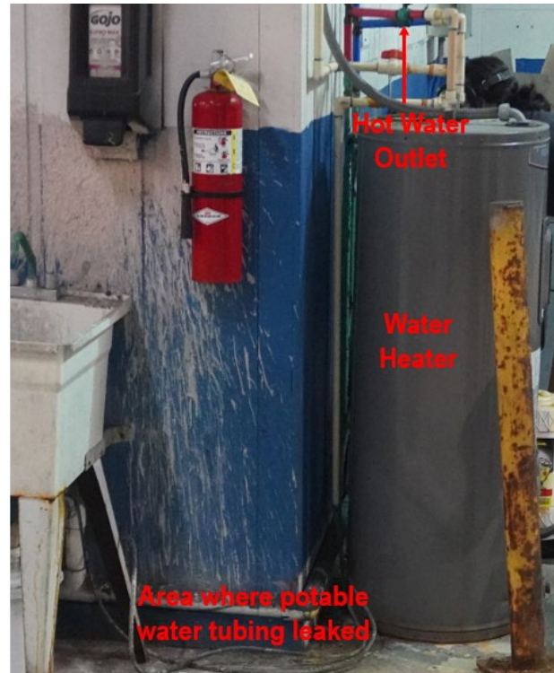
Figure 24. Location of polyethylene line that leaked, causing an area in the Bio-Lab Conyers Plant 6 to flood. (Credit: CSB)
