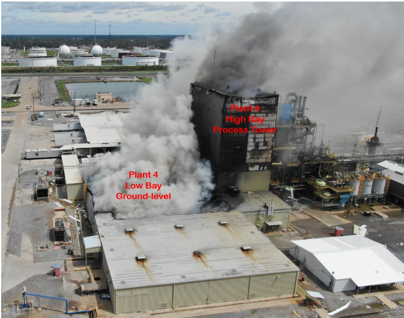
Figure 9. Decomposing chemicals in Plant 4 on August 27, 2020. (Credit: Louisiana State Police, annotations by CSB)
