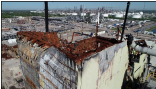
Upper 35' of tower looking NW, after fire & demo work (Atlas UAV, 9/30/2020)
