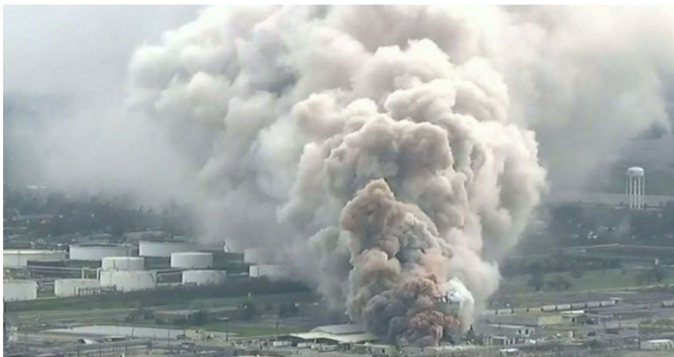
Figure 7. Photo of decomposition gases, including toxic chlorine, released from Bio-Lab Plant 4 after the building was severely damaged during Hurricane Laura and rainwater contacted the stored chemicals. (Credit: The Associated Press [22])
