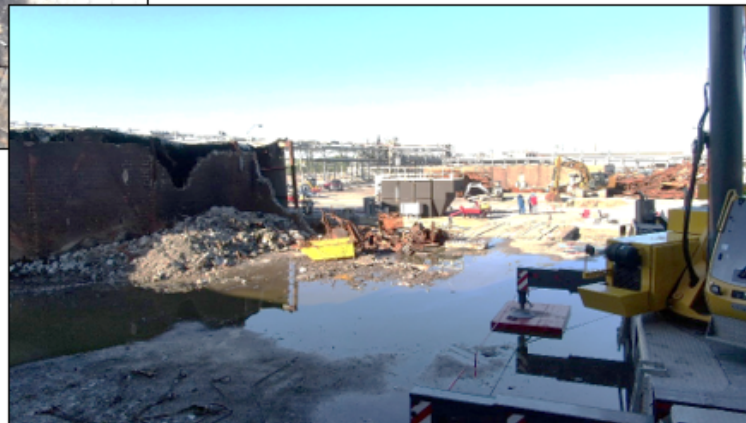
View looking west (Atlas UAV, 9/30/2020)
