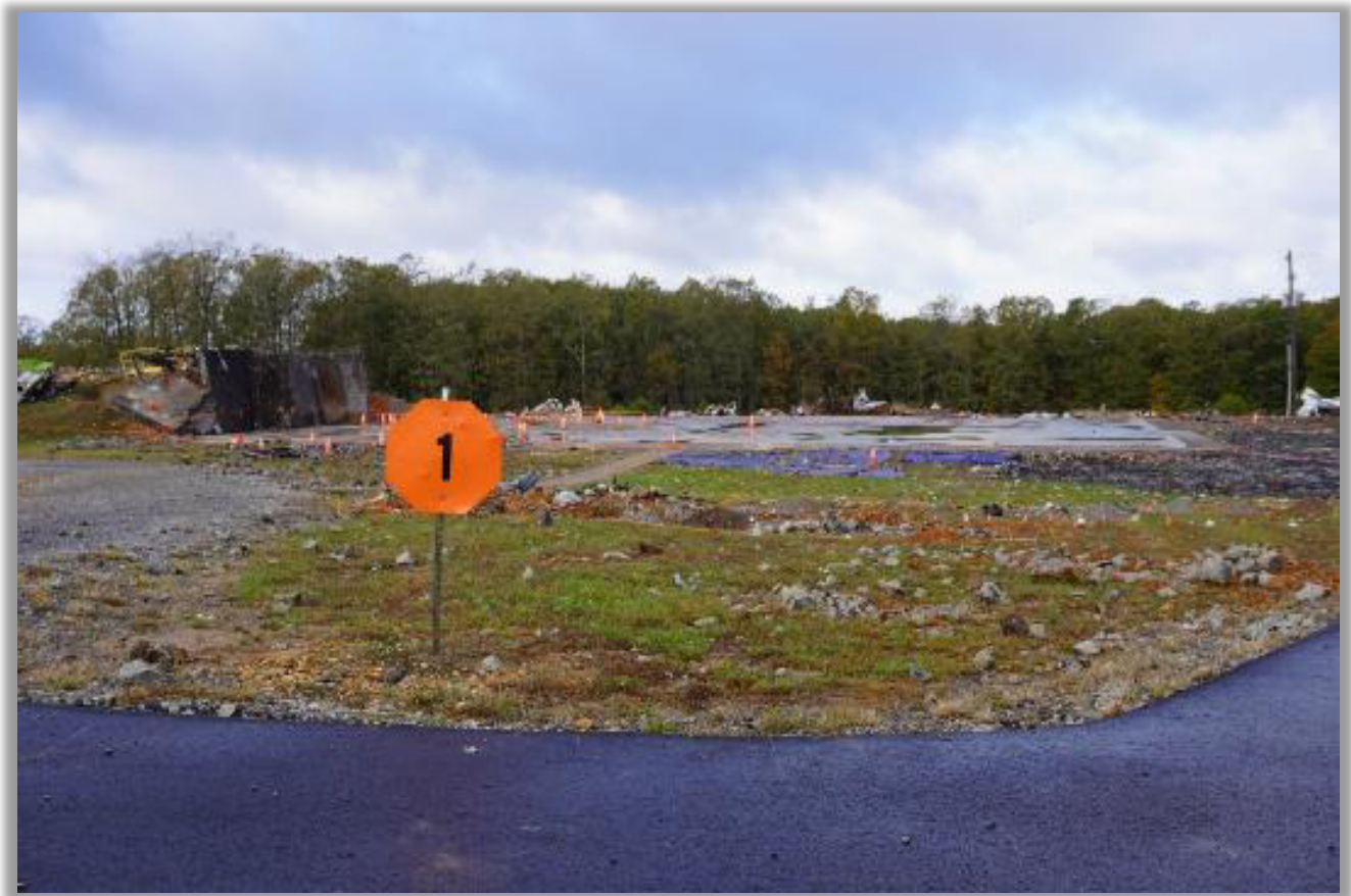
Figure 10. Post-incident photo of the Building 602 location after the foundation was cleared. a (Credit: CSB)
