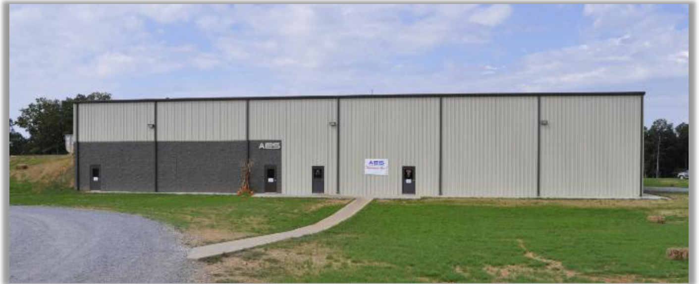
Figure 2. Pre-incident photo of Building 602. (Credit: AES)
