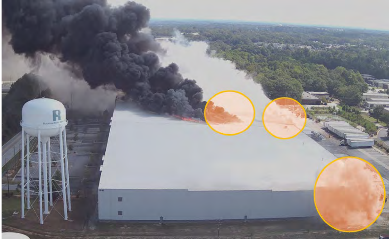
Figure 43. Aerial shot of the second building fire at Bio-Lab Conyers 12 Storage Warehouse on September 29, 2024, resulting from the multiple-point heat source generated by decomposing oxidizers and combustible materials. (Credit: RCFR, annotated by CSB)
